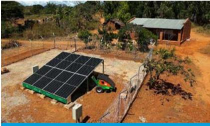
The combined use of solar panels and storage (the microgrid) enables remote power
